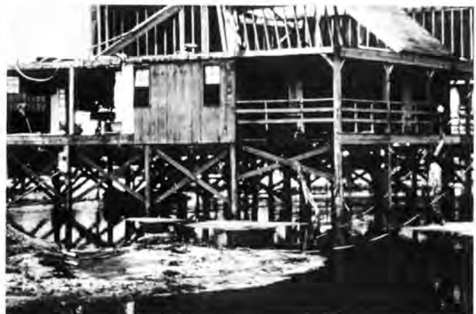
Figure 4.23. Diagonal Bracing
