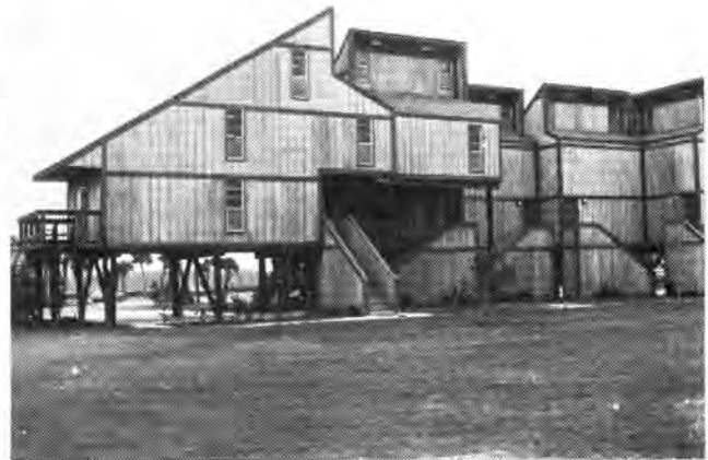
Figure 4.4. Elevation by Posts
