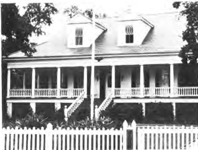
Figure 4.15. Pier Foundations
