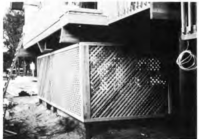
Figure 4.54. Breakaway Walls
